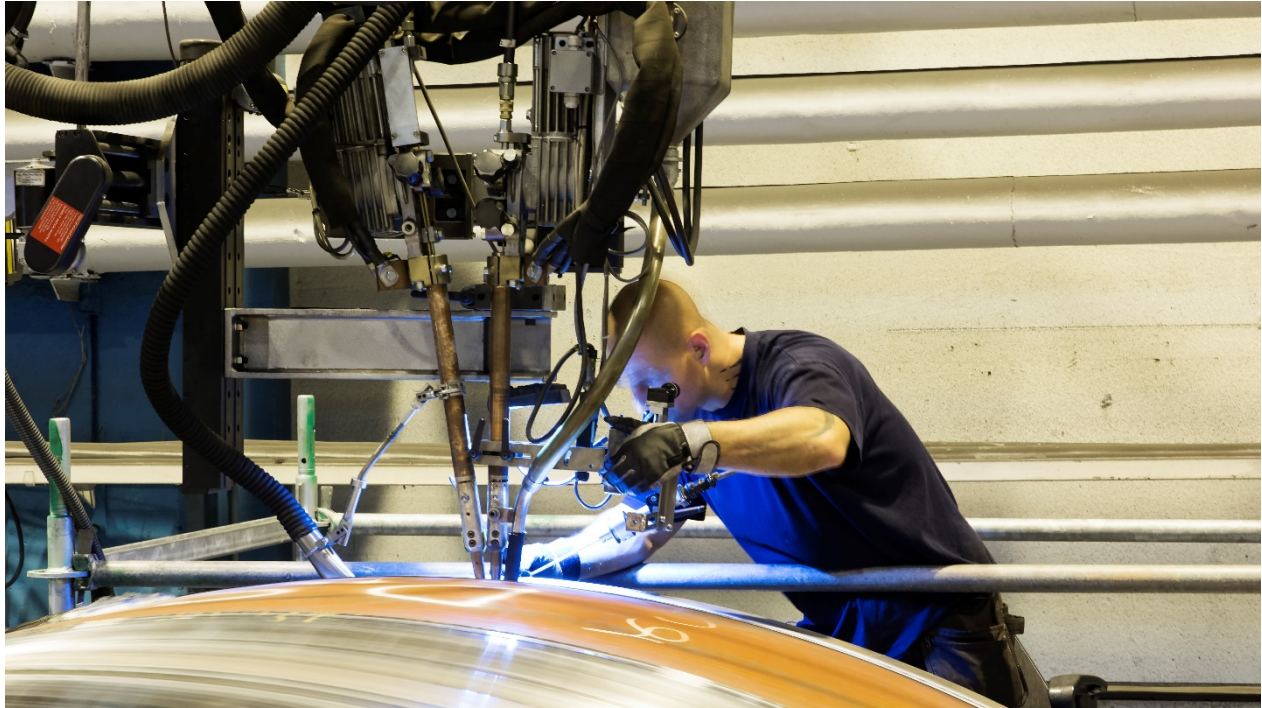
Figure 5. Assembly welding of steel yankee dryer.
