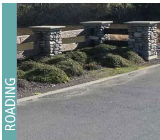
Chip seal + flush concrete edge
