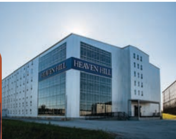
One of Heaven Hill's 61 warehouses.
