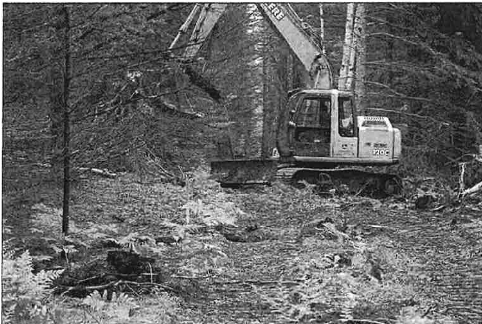
Photograph 6: Proposed Runway at Station 1+150 looking south.
