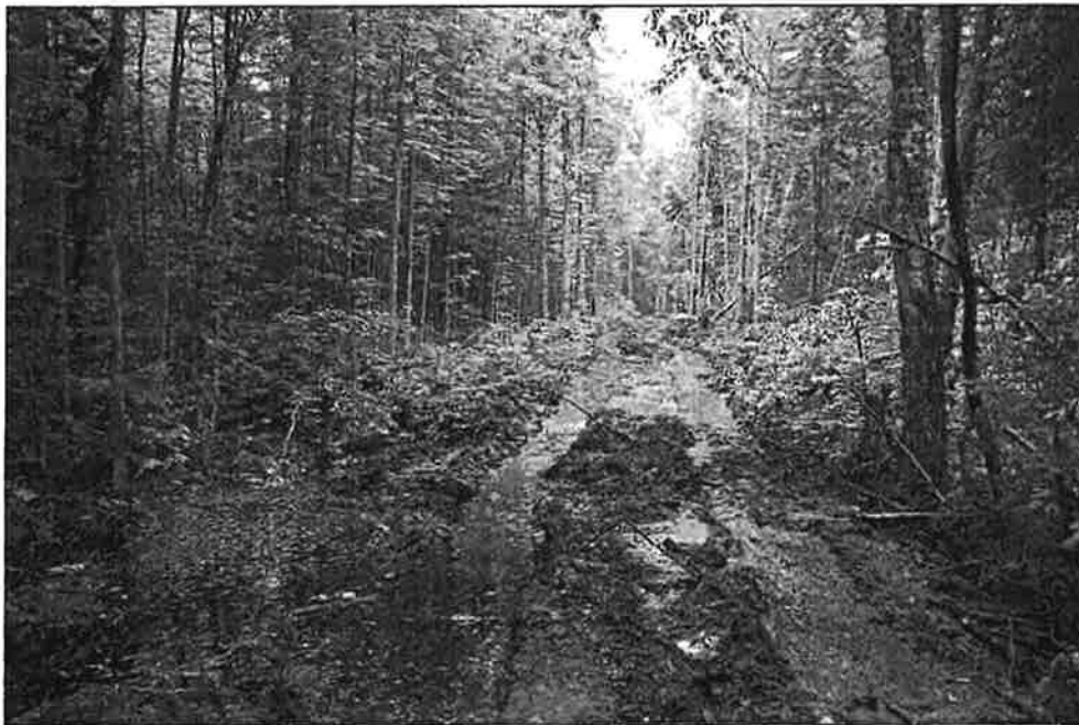
Photograph 9: Proposed Runway at Station 1+700 looking south.
