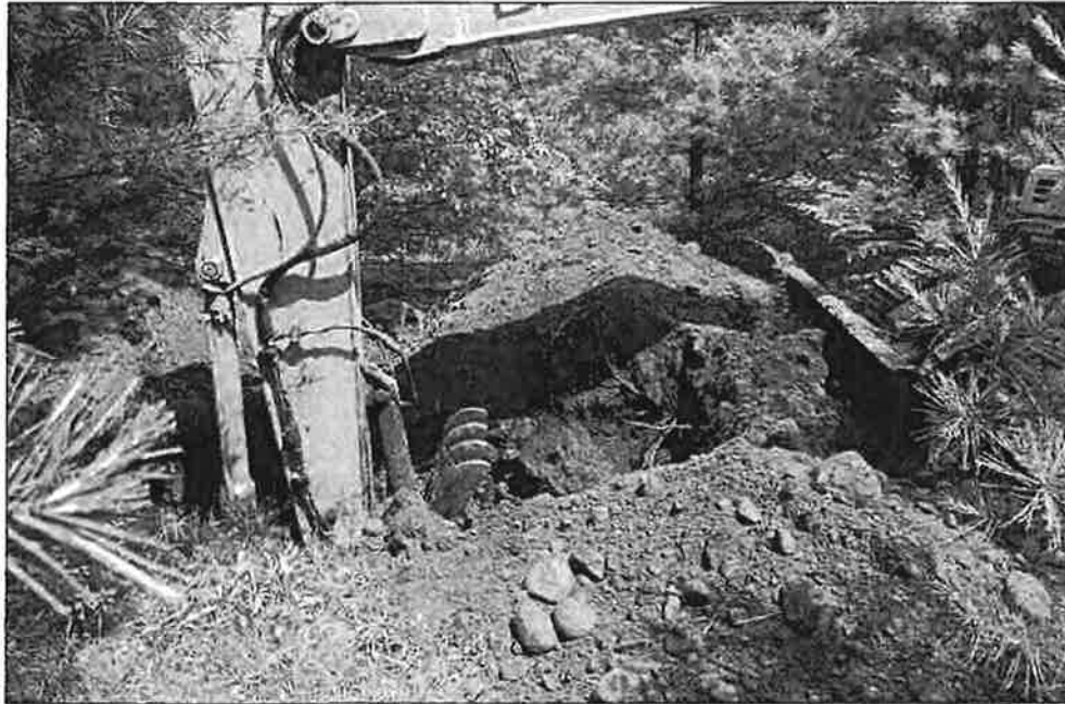
Photograph 14: Typical soil conditions in test pit 240.
