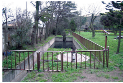
▲ Taoyuan Wires and Cables Plant waste treatment facility
