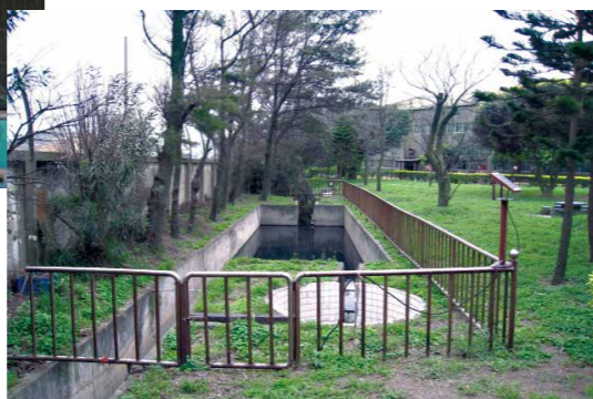
Taoyuan Wires and Cables Plant waste water treatment facility
