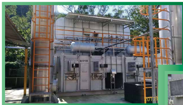
3P Program on-site audit(1/2)
