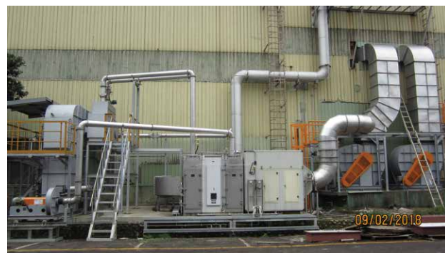
RTO in Tayuan Plant (under construction)
