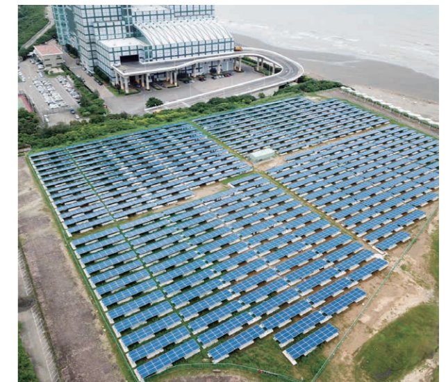
▲ PV roofing on Kanhai Park's public buildings
