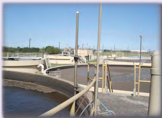
Wastewater Treatment Facility
