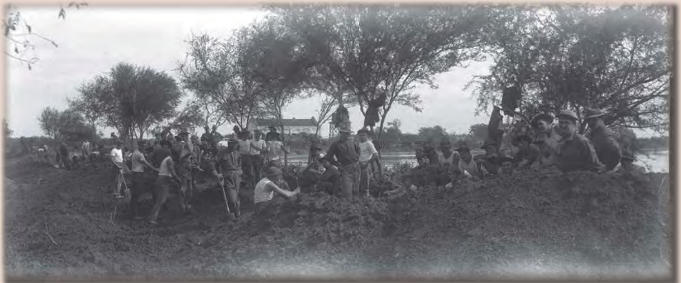
Soldiers working on levee, circa 1917
