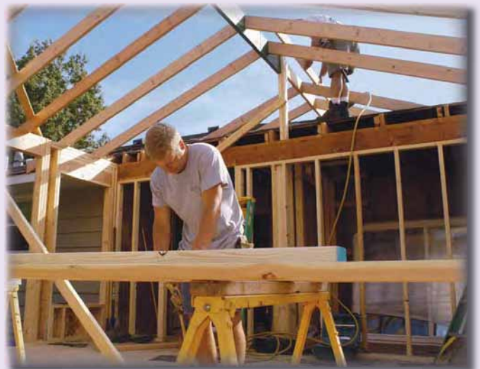
New home construction
