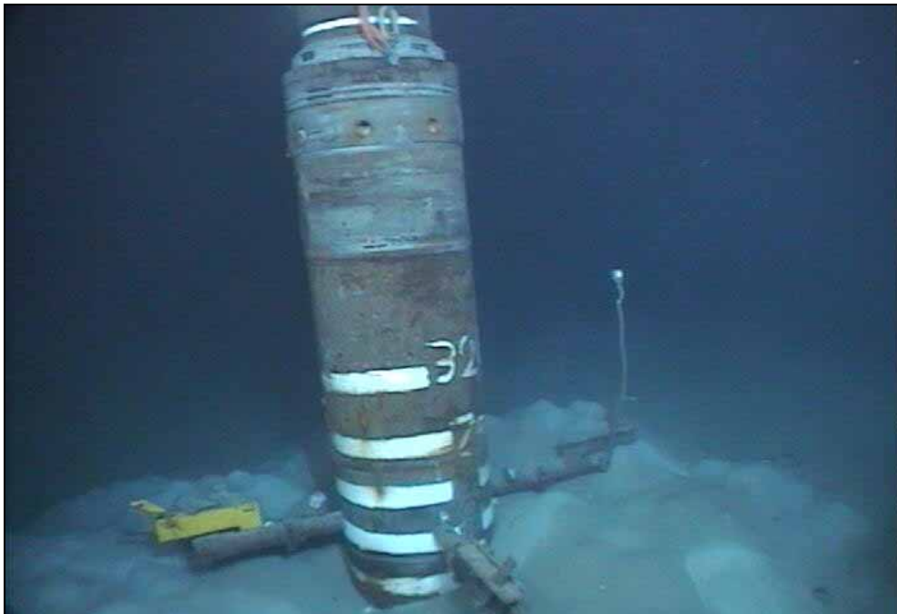
Figure 7-62. Chevron wellhead observed during D282, AC818.
