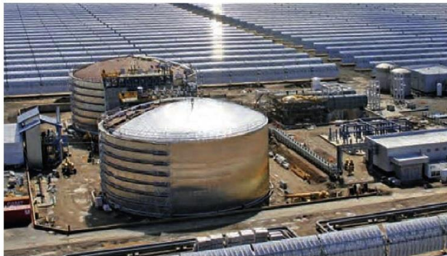
Figure V-4: A molten salt TES pilot plant located in Seville (Spain) [58]
