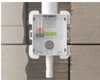
Put the siphon into the wall niche
