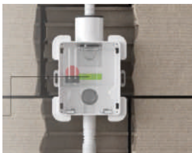
Connect the pipes. Check horizontal level
