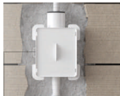
Protect the siphon by applying the protection cover
