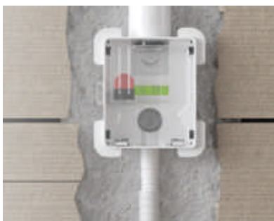
Plaster the wall niche
