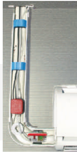
LAYING PIPES AND PUMP
