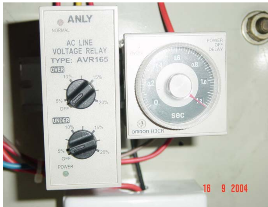
Figure 26: Changing the Voltage threshold and time delay
