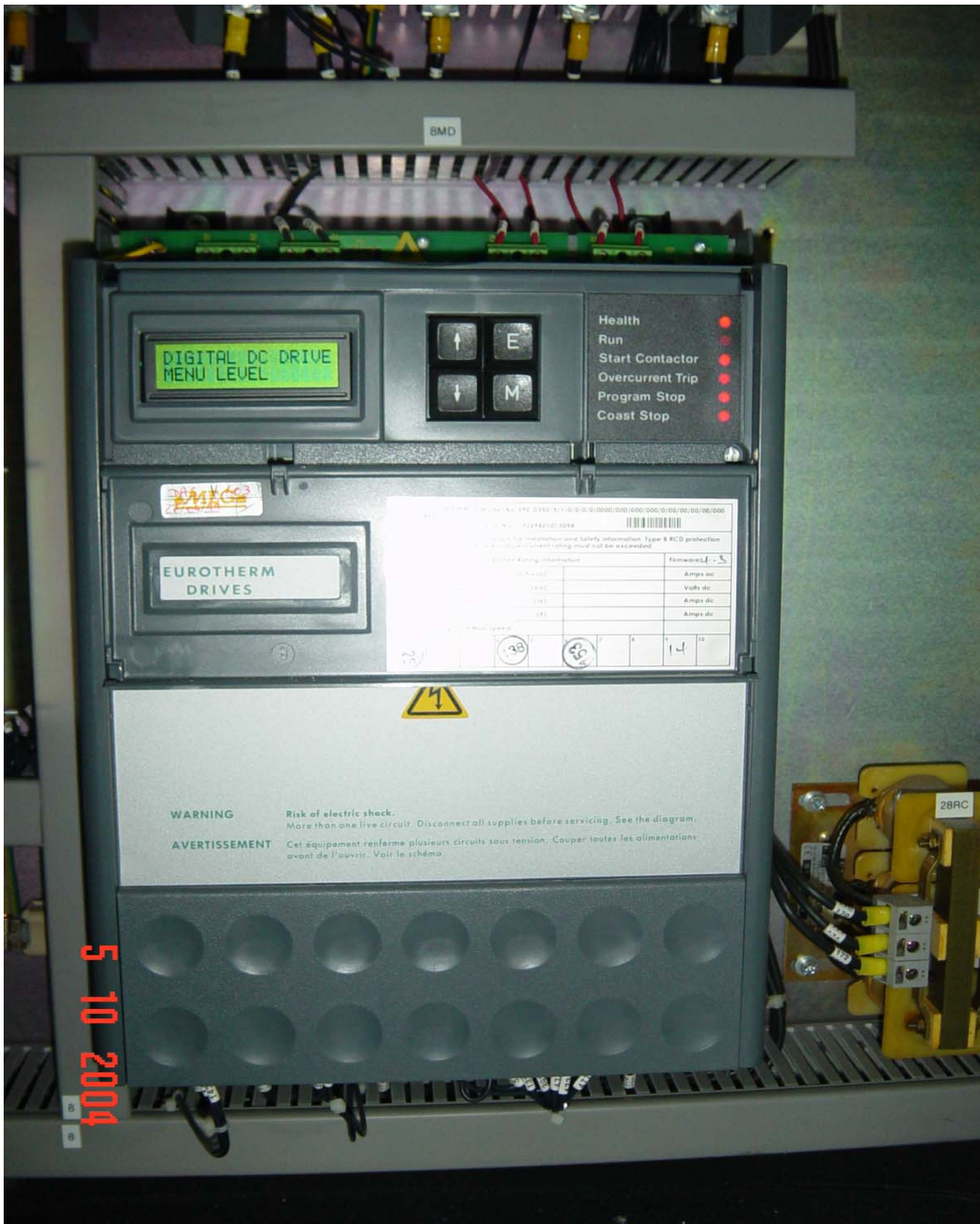
Figure 19: Direct current (DC) drive
