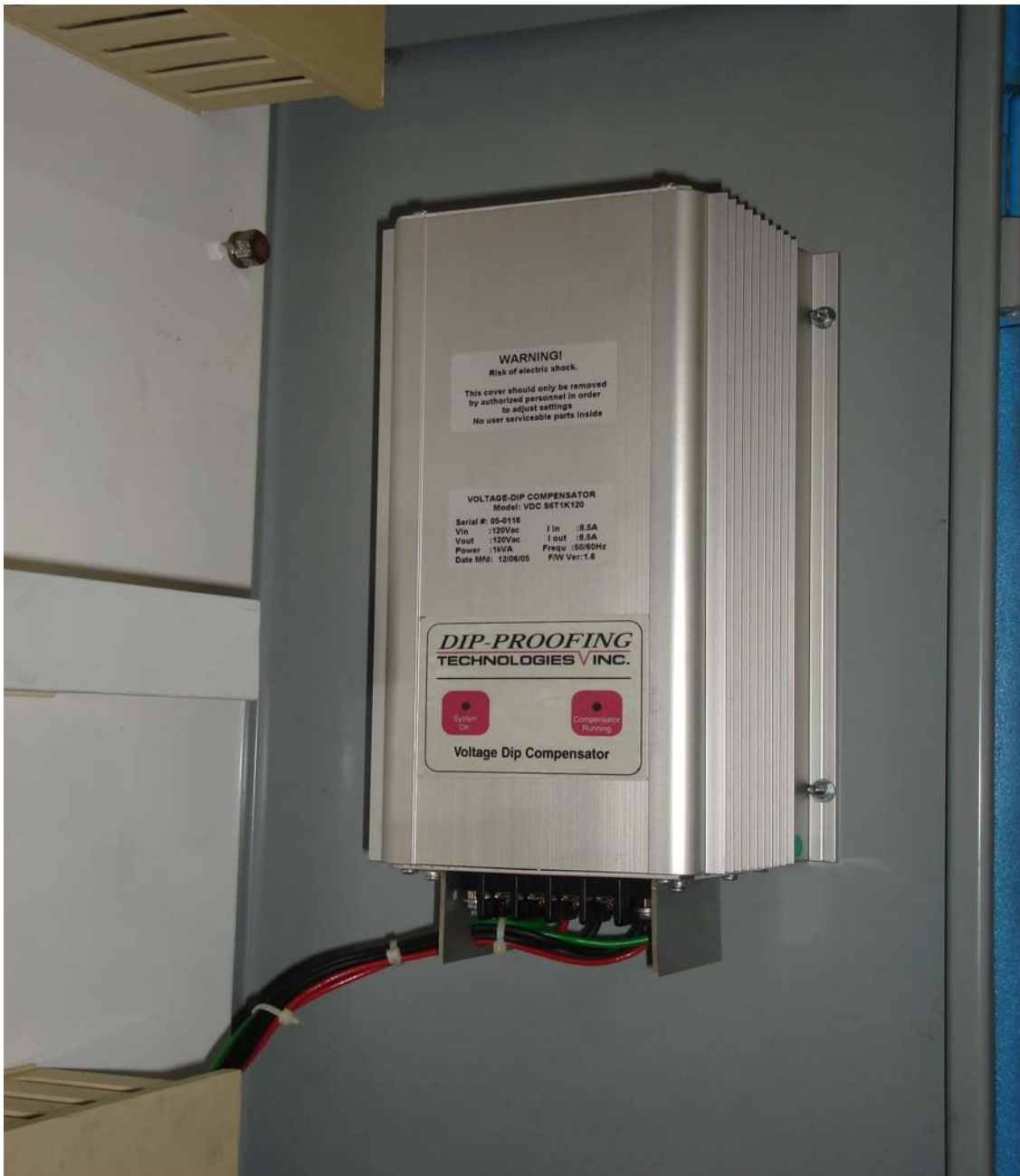
Figure 33: Voltage Dip Compensator (VDC)
