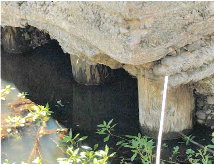
Photo 3-19: Wooden Piles Supporting Cultural Resources Site Number ARP18-1's Southwest Pier.
