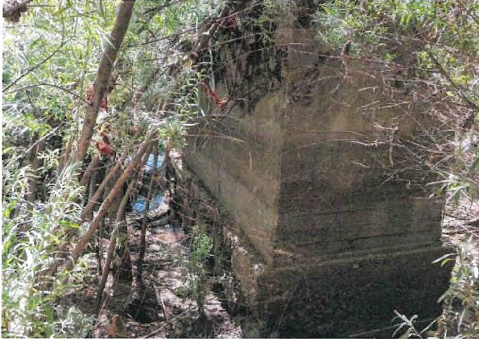
Photo 3-16: Cultural Resources Site Number ARP18-1 Northeast Pier.
