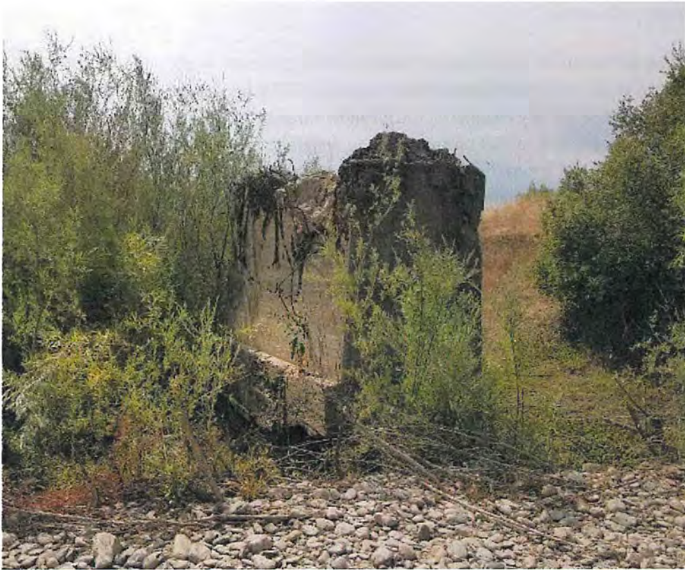
Photo 2-3: Existing historical bridge abutment.
