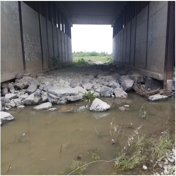
Photo 2-7: Existing concrete and rock between two bridge bents under the Antelope Boulevard/Highway 36 Bridge.
