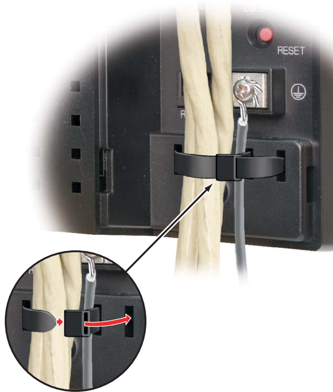
Figure 11: Securing the Cables
