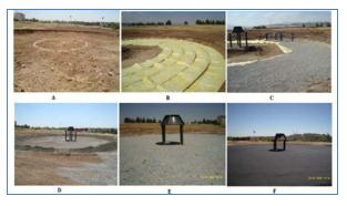
Fig. 6. Pictures showing the construction steps of ground of the Abdulceli prototype (A ground floor, B Aluminum folio with glass wool, C Gravel laying, D Sand, E Glass laying, F Asphalt paved) [11].
