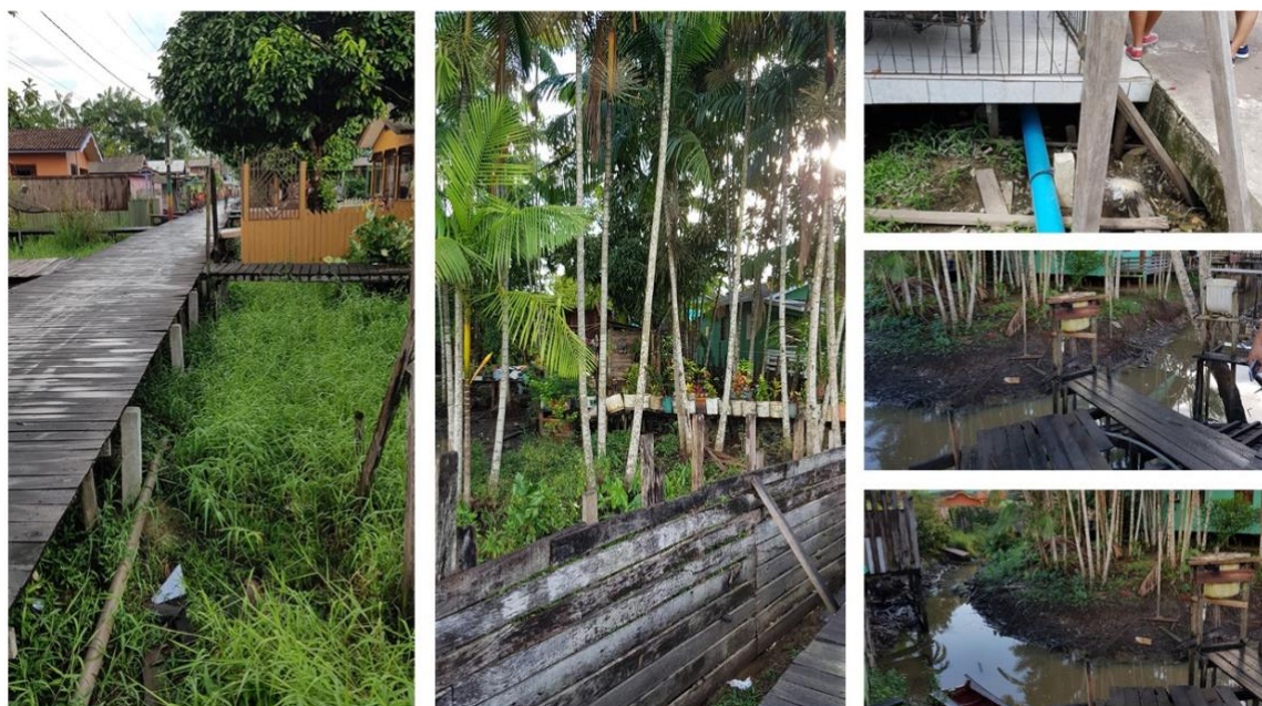
3 4 Figure 2. Infrastructure deficit in the city of Afuá, Pará, Brazil (Source: Laboratório de Estudo 5 das Cidades Collection/UNIVAP) .
