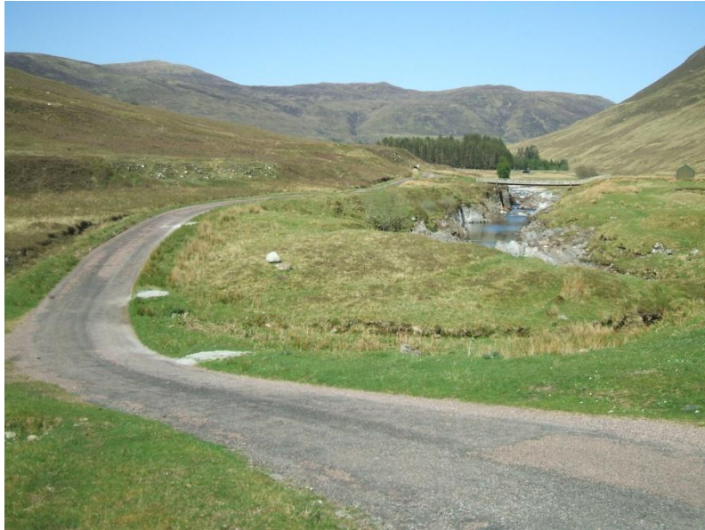
View to the wooden bridge with the stones left of centre.
