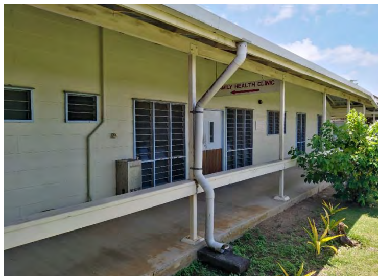
Photo 20. The new wing built on the site of the old DDT Storage Shed
