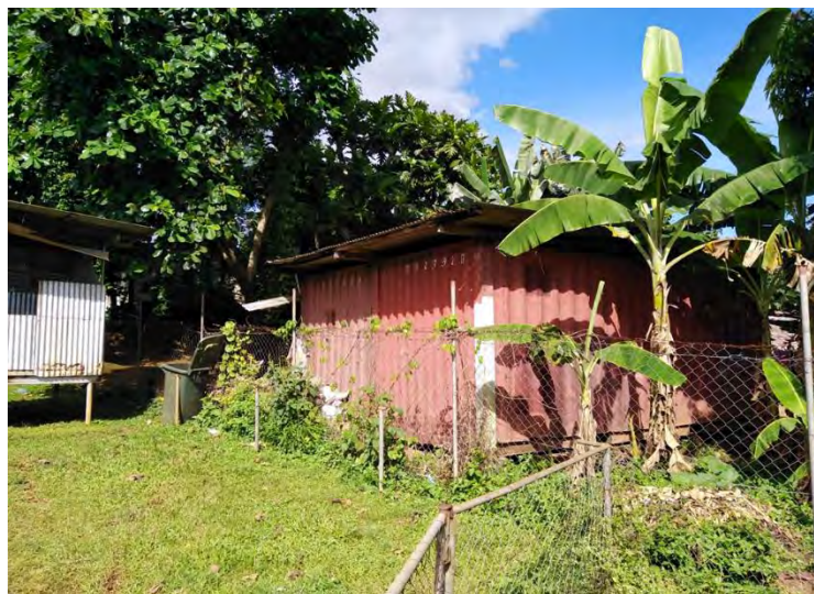
Photo 18. The 2 x 20ft containers that once contained the old DDT stocks
