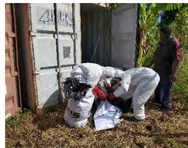
Photo 12. Safeguarding work – double bagging
