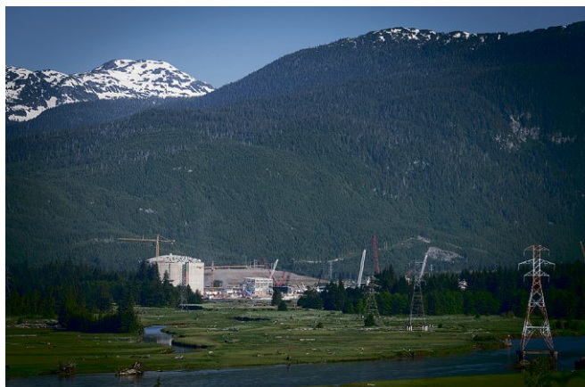
◀ Across the Kitimat River is LNG Canada's natural gas storage tank, which will be one of the largest in the world, at 225,000 cubic metres
