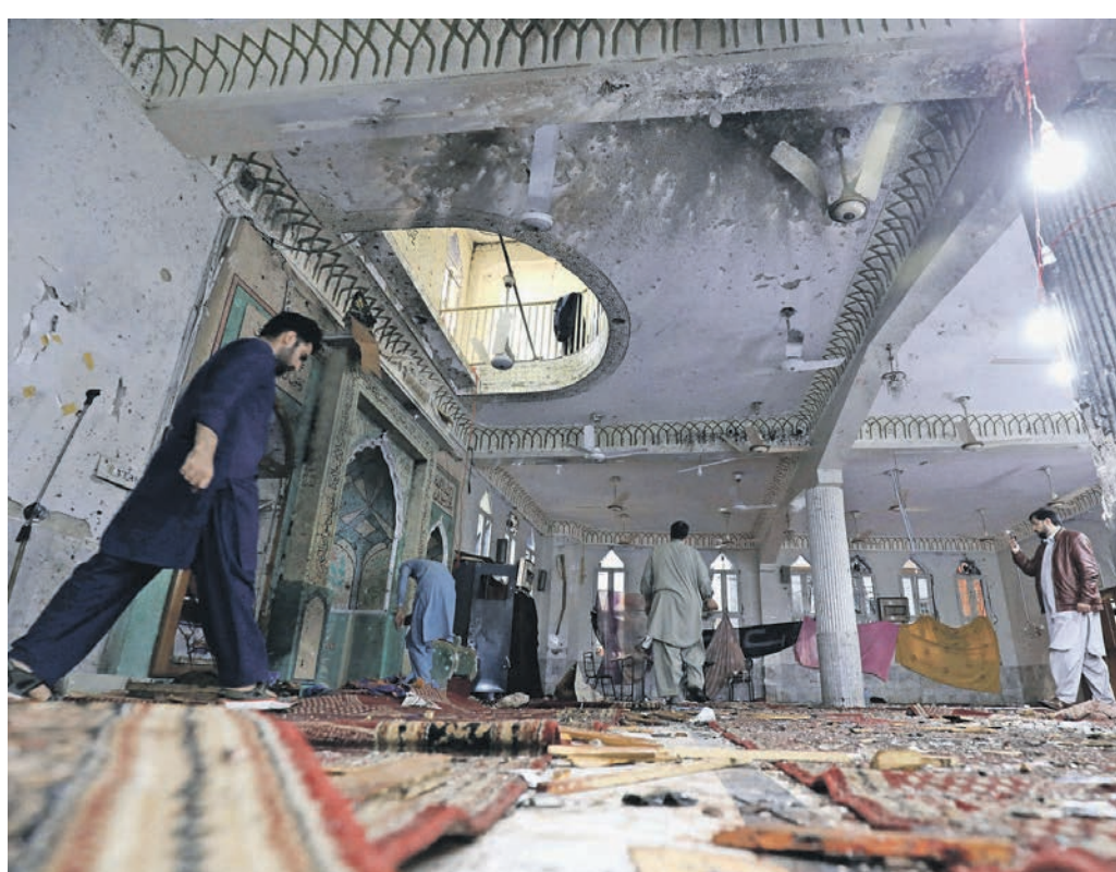
Investigators survey damage at the Kucha Risaldar Shia Mosque's prayer hall in Peshawar, Pakistan, after a suicide bomber attacked Friday with a crude, ball-bearing-laden device. FAYAZ AZIZ/REUTERS
