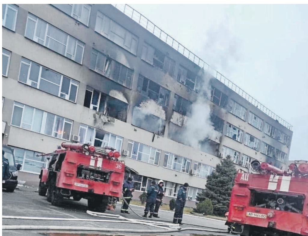
Smoke rises on Friday from a badly damaged training building hit by a projectile near the reactor complex at the Zaporizhzhia Nuclear Power Station in southern Ukraine. Russian forces now control the site.
