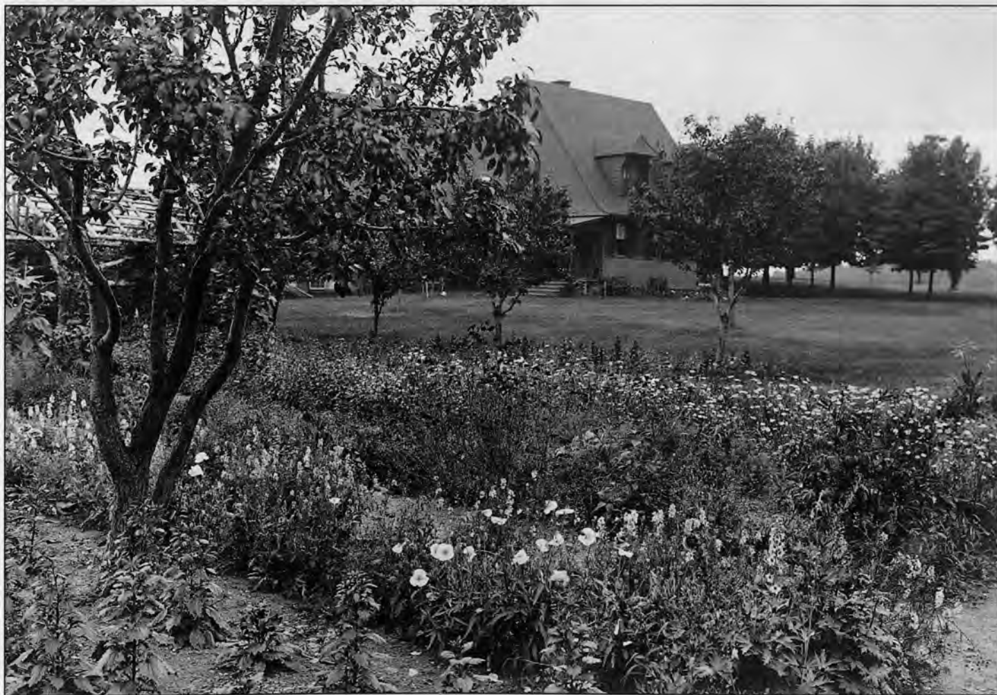
View of stable and lodge from garden, 1905.
