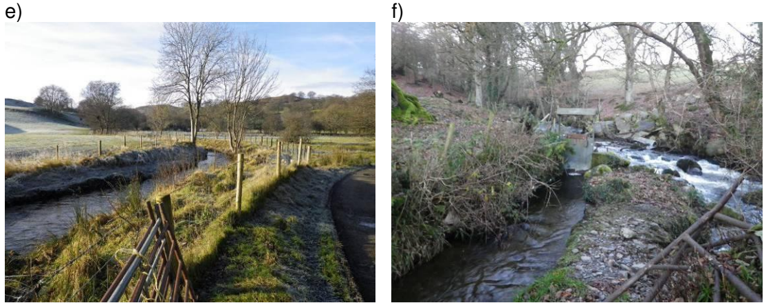
Figure 5.8 a) Weir for water supply; b) managed water access point for livestock; c) bank protection on outside of bend; d) straightened section; e) embanked section (probably using spoil taken from new course) and f) sluice for domestic hydropower scheme, Afon Meloch
