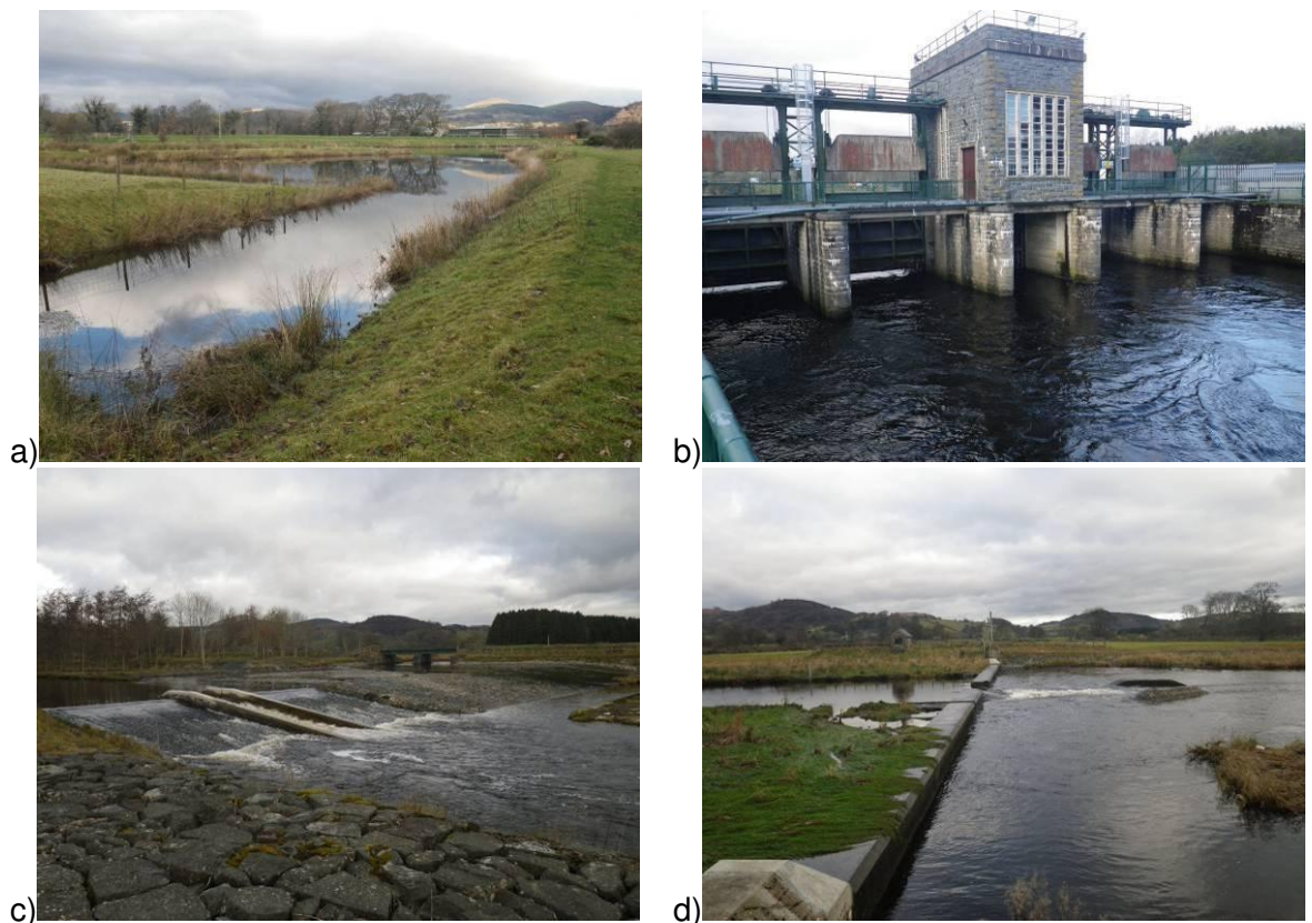
Figure 5.11 Structures at Treweryn confluence; a) Side channel right bank probably for flood storage, b) Sluice gate to control flow rate in Dee c) Salmon Steps and d) Weir by Bala Enterprise park
