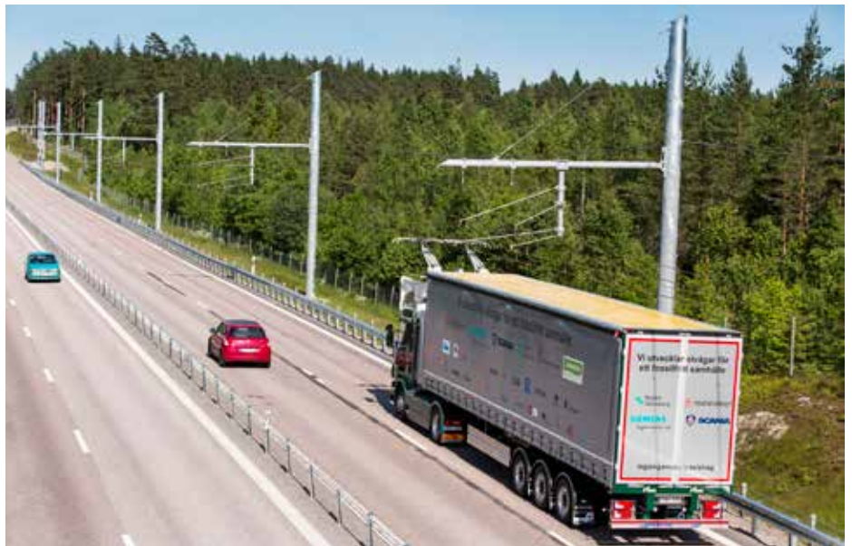
Elväg E16. Installation of the rail on eRoadArlanda.
