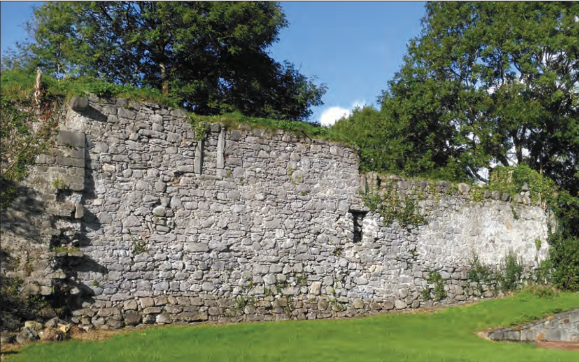
Illus. 1.13—Tell-tale signs in the masonry of Moycullen Castle suggest that it was originally of Anglo-Norman construction, remodelled by the Gaelic O'Flahertys in the 14th century. (Hugh Gallagher)
