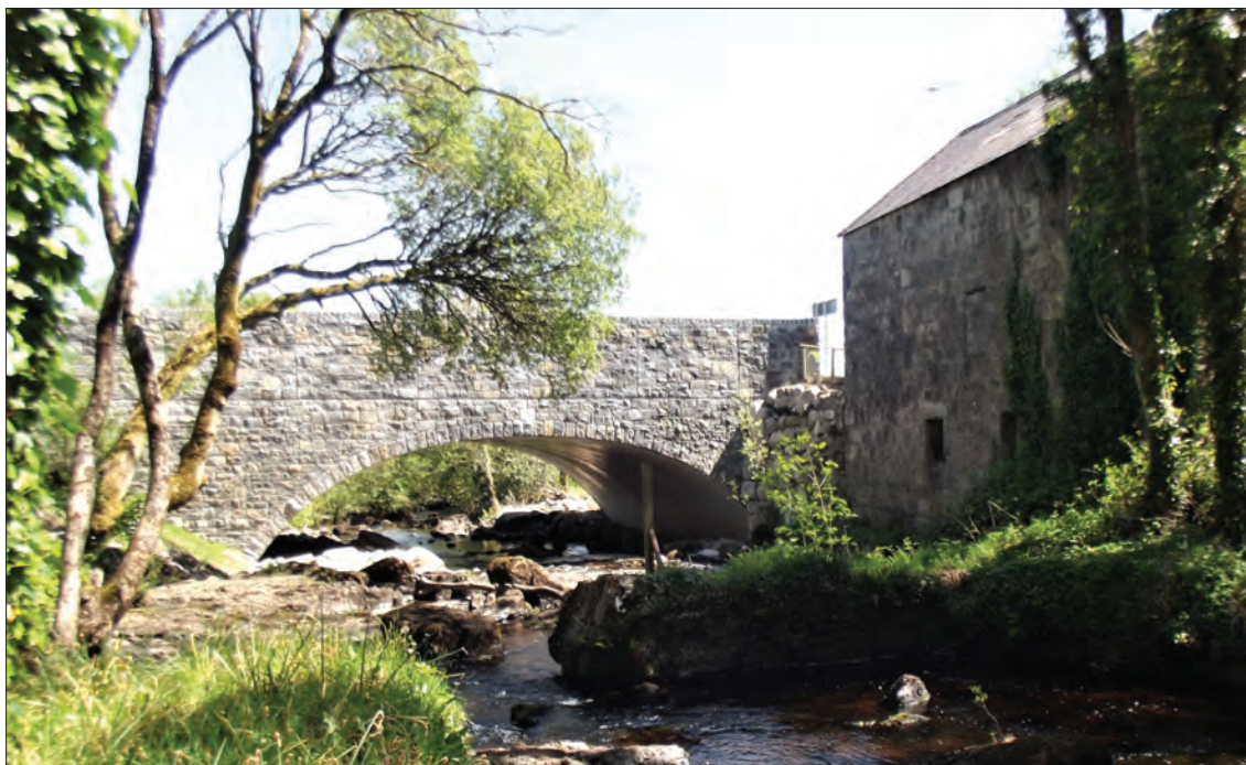
Illus. 1.32—The old Clydagh Bridge and the adjacent Victorian grain mill formed a pleasing rustic group on the Lough Kip River. The new bridge is a much bigger structure but its stone cladding attempts to capture some of the original character of the place.
