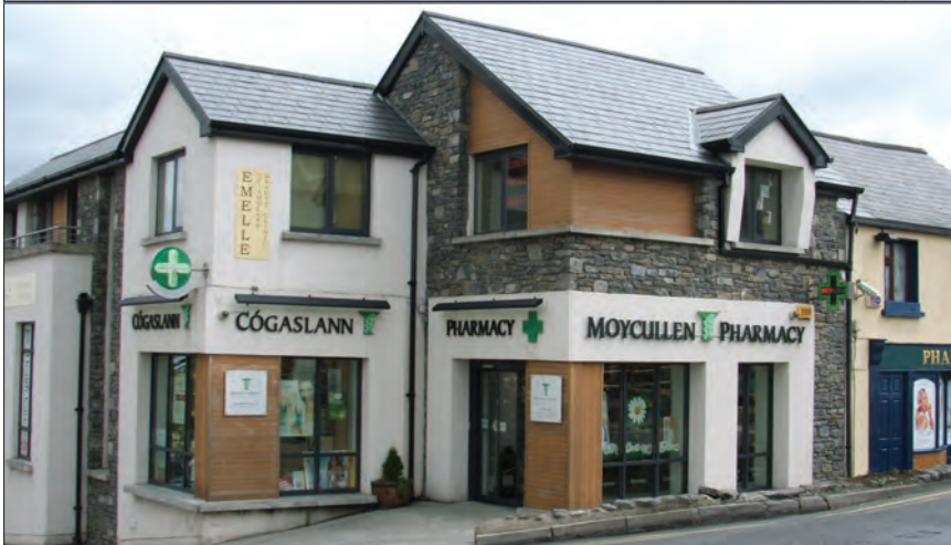
Illus. 1.28— Some recent commercial developments in Moycullen have sought to replicate the scale and fabric of older shopfronts (above); others mix old and new materials in the same design (below).
