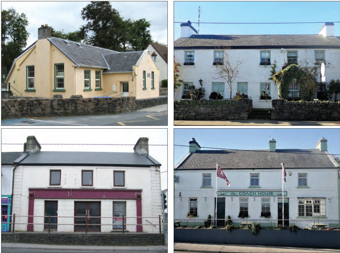
Illus. 1.24—Several buildings in the village recall the social and economic life of early modern Moycullen. Árus Uilinn was once a National School (top left); the White Gables occupies the former RIC station (top right); Morrisons' House was used for Church of Ireland worship (below left); and Fox's Bar (now the Coach House) doubled as a ticket office for Bianconi cars and for the Cunard White Star shipping line.
