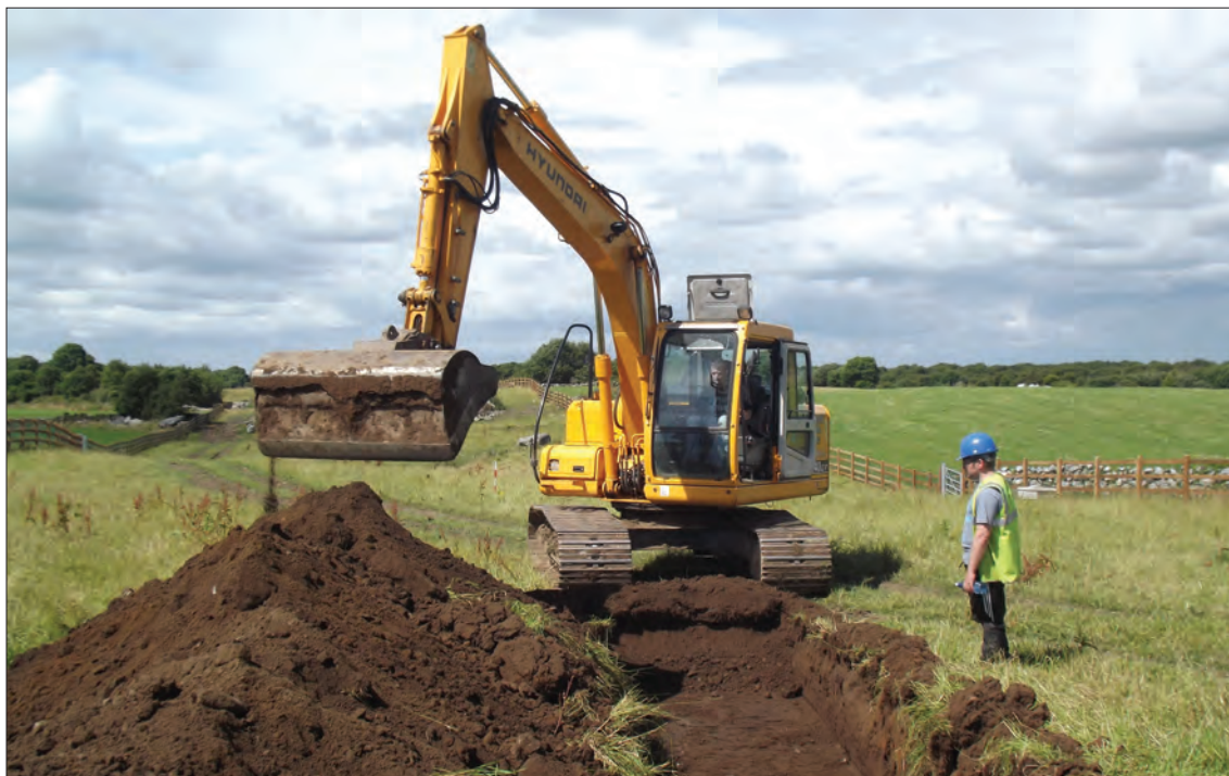
Illus. 2.1—Test excavations were opened by machine, under archaeological supervision, throughout the footprint of the bypass.
