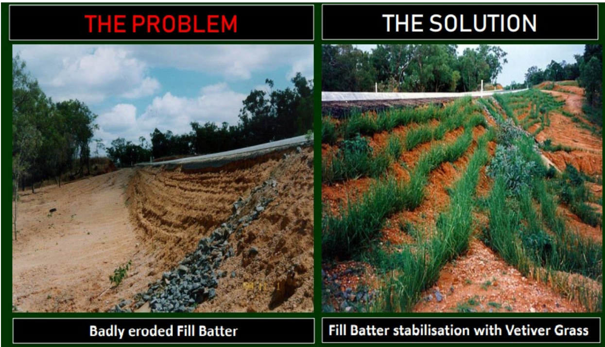
Figure 9 - 6. Shows the Vetiver grass function in protecting the soil erosion.
