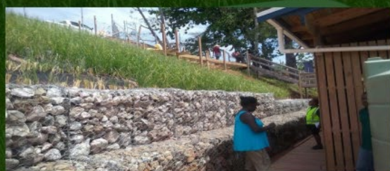
Figure 9 - 7. Shows the Vetiver grass planted as Dam Wall Stabilizer and helps protect the gabions from erosion.
