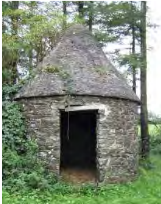
Old powder house (explosive store) at Earlishill, Slieve Ardagh Coalfield, Co. Tipperary
