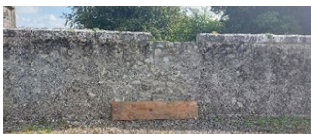
Loughkeen Church Boundary Wall -before/after
