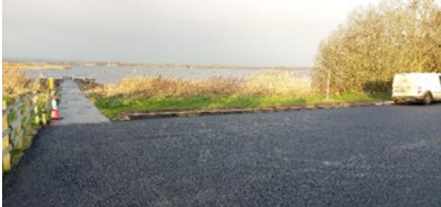
Resurfacing works at Mota Quay
