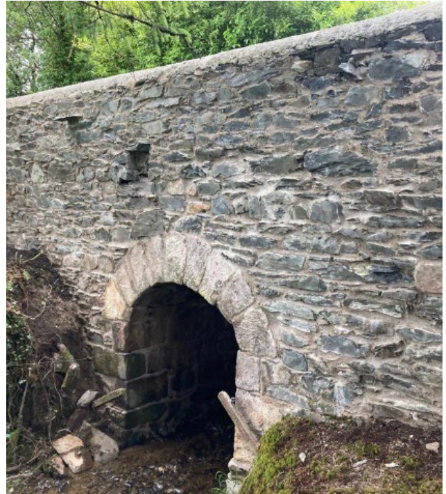
Remedial Works at Shanballyedmond Bridge, Rearcross
