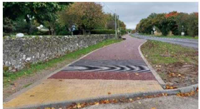
Riverstown resurfacing & footpath works
