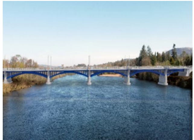
Shannon Bridge Crossing
