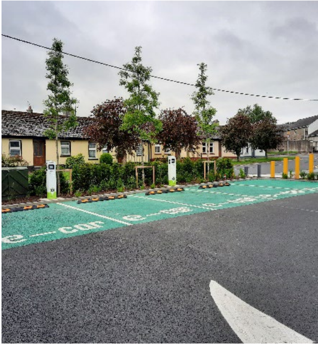
EV Charging Points -John's Lane Car Park
