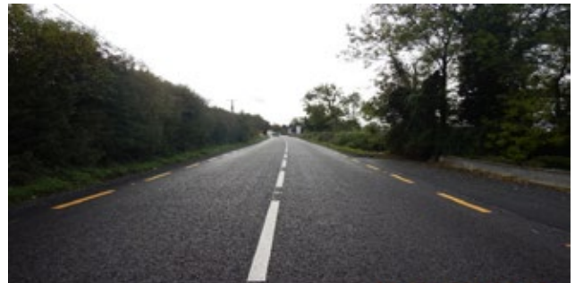
N62 Kilnoe (M8) Pavement Scheme
