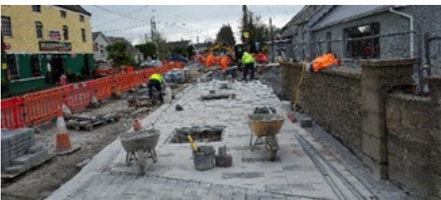
N76 Grangemockler works in progress
