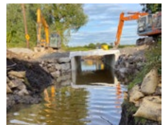
Bridge Rehabilitation Works at Kilclonagh, Moyne
