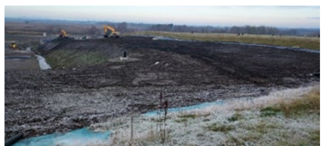
Ballaghveny Landfill - Wedge Cell being filled with waste 13th December 2022
