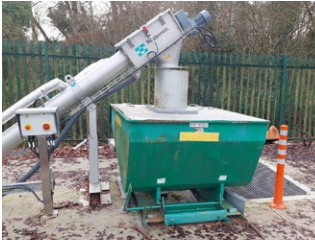
Puckane Wastewater Treatment Plant Upgrade
