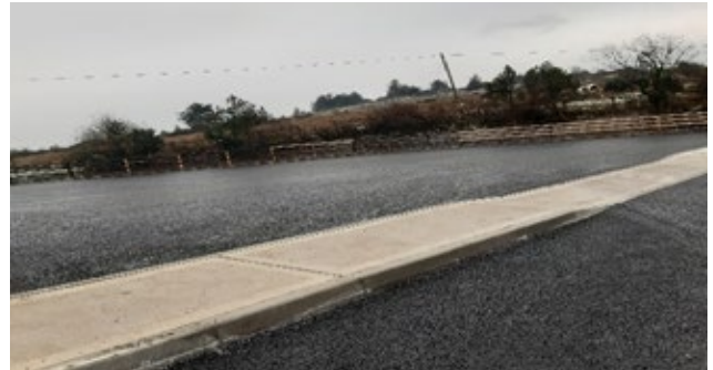
Resurfacing works at Steppe Car Park
