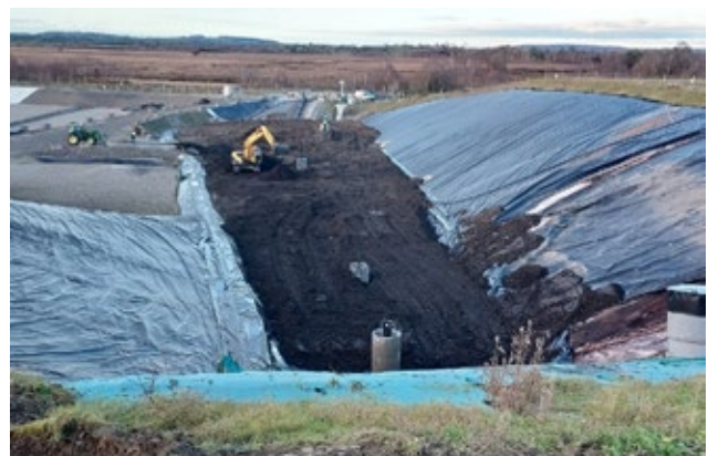
Ballaghveny Landfill - Wedge Cell being filled with waste, 15th December 2021
