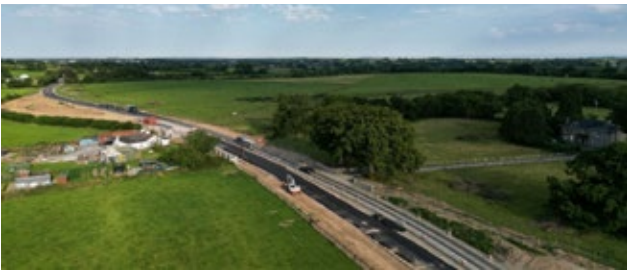
N74 Ballyhusty during construction in 2022
