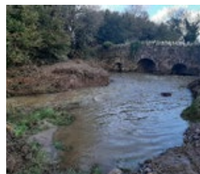
Bridge on Lingaun River at Brenormore near Slievenamon
