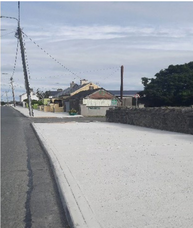
Footpath Improvement Works at Cloughjordan
