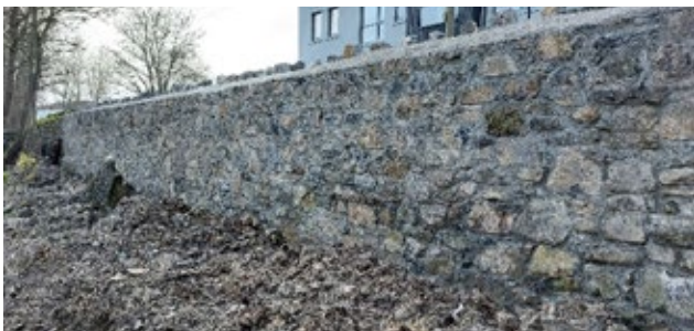
Repair of Stone Wall at Borrisokane Community Park
