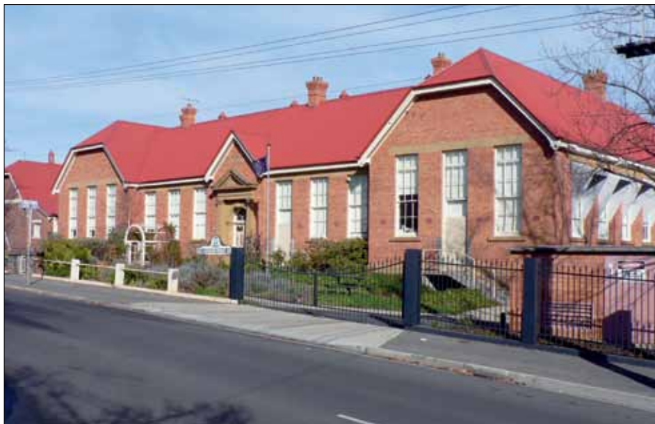
Fig. 12. East Launceston Primary School in 2013, designed by Orlando Baker in 1906–07 as the ‘East Launceston Public School’.
