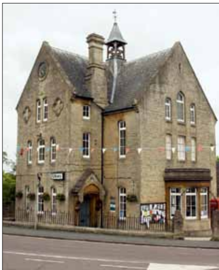
Fig. 2. Workmen's Institute, Purton (now the town library). Designed by Orlando Baker and constructed over 1879–80.
