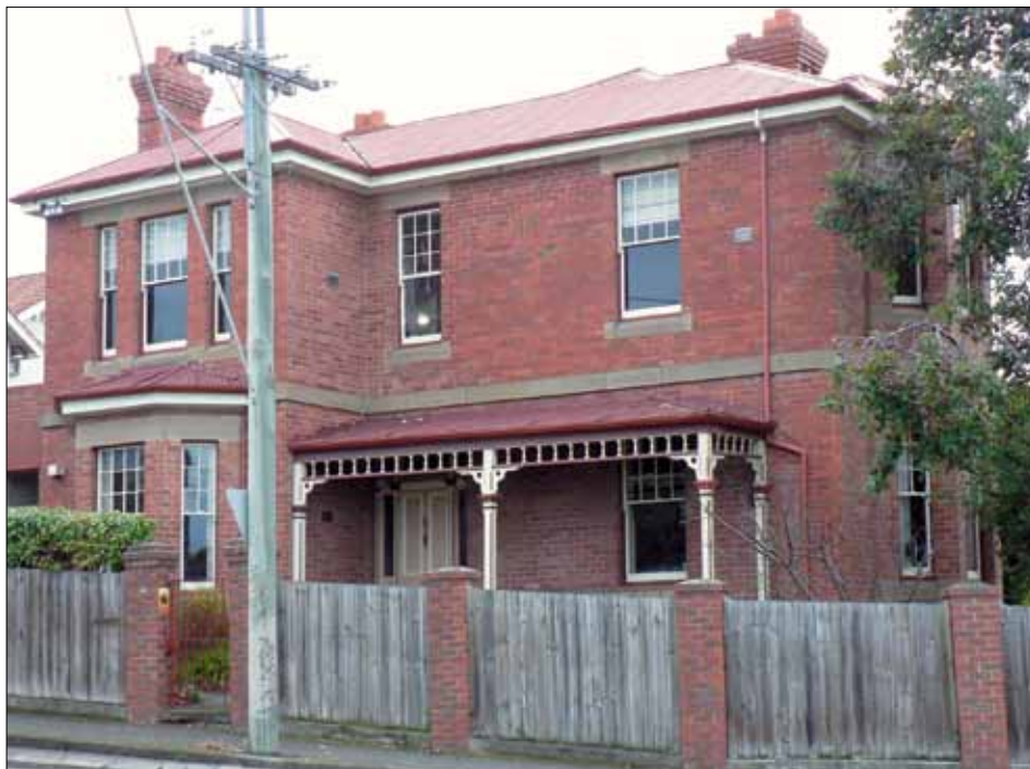
Fig. 14. Orlando Baker's home – Glenville – on the corner of King and Parliament streets, Sandy Bay. Constructed over the period c. 1908–10, it represents the only known example of his private design work in Tasmania. Originally 70 'King Street West', its number was changed to 96 in 1914 and remains the same today.
