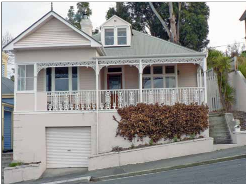
Fig. 5. The house at 60 (now 72) Barrack Street occupied by Orlando Baker from early 1893 until late 1909 or early 1910. The forward-jutting Federation-era extension on the left, with the gabled roof, is unlikely to have been added during his tenancy. It represents only a small addition to the original frontage, and seems to date from the period 1910–18 (see endnote 41).
