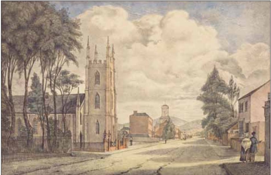
Fig. 7. H.G. Eaton, St Joseph's Church Macquarie Street, Hobart Town, T. Bluett, Hobart, 1844. The neighbourhood of the Tilley's foundry and residence on the corner of Macquarie and Harrington streets, Hobart. The building visible on the extreme right is likely to be the foundry or house.
