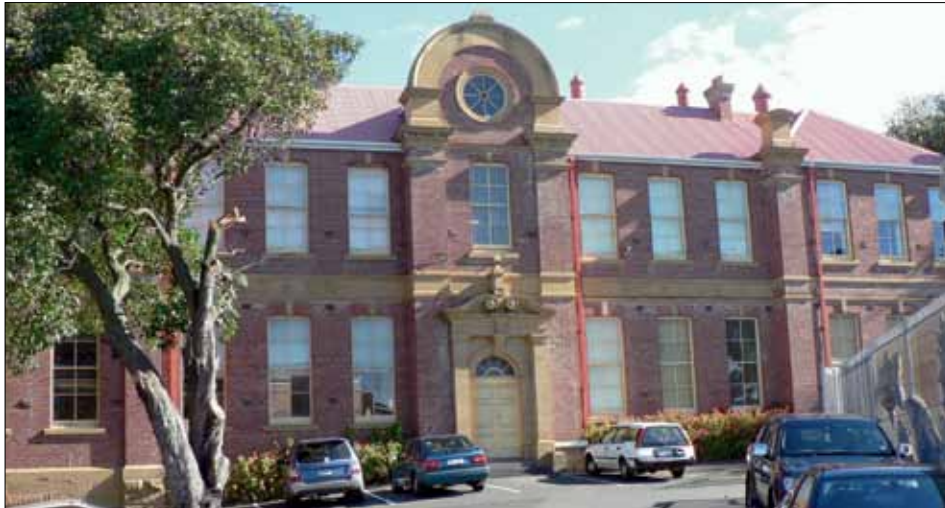
Fig. 15. Front view of the Elizabeth Street School building, designed by Orlando Baker in 1909 and now part of the Elizabeth College complex.
