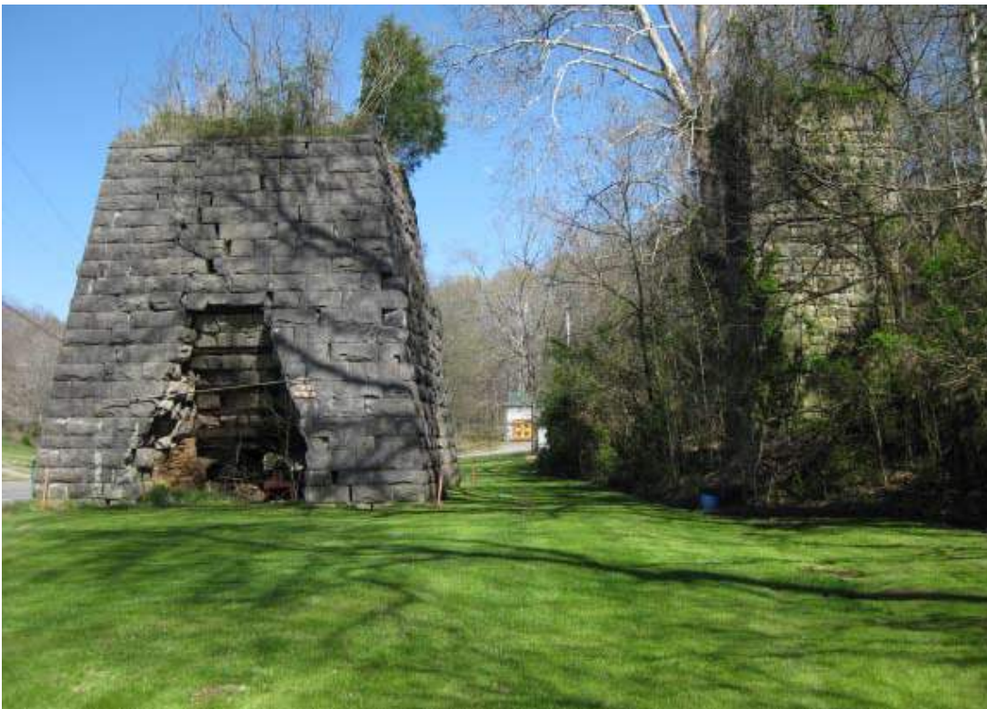
Furnace stack (l) and charging bridge (r)
