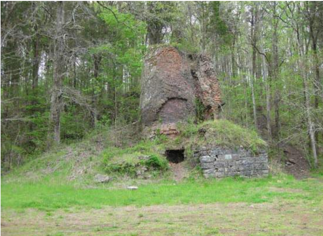
Remains of furnace stack, facing east
