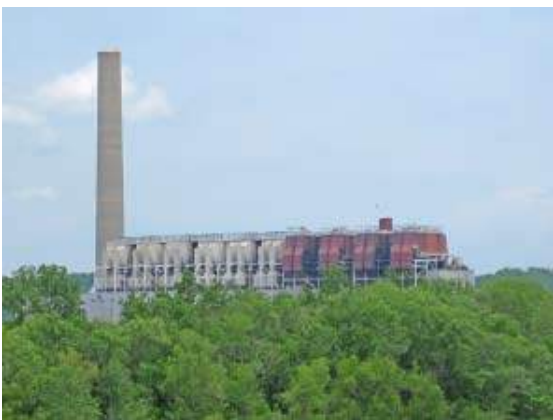
Johnsonville Steam Plant
