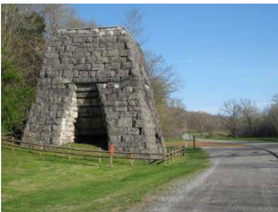
Furnace stack, facing south
