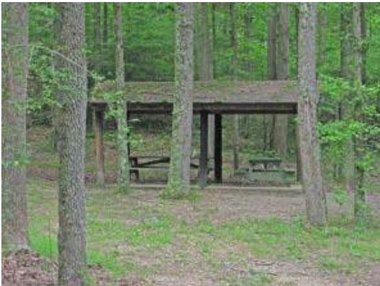
Rustic shelter in picnic area, Nathan Bedford Forrest Park
