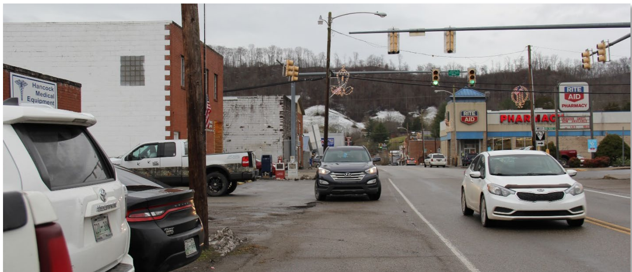
This portion of SR 33 / Main Street (near the Post Office) illustrates an example of where the paved shoulder tapers into private business parking areas.
