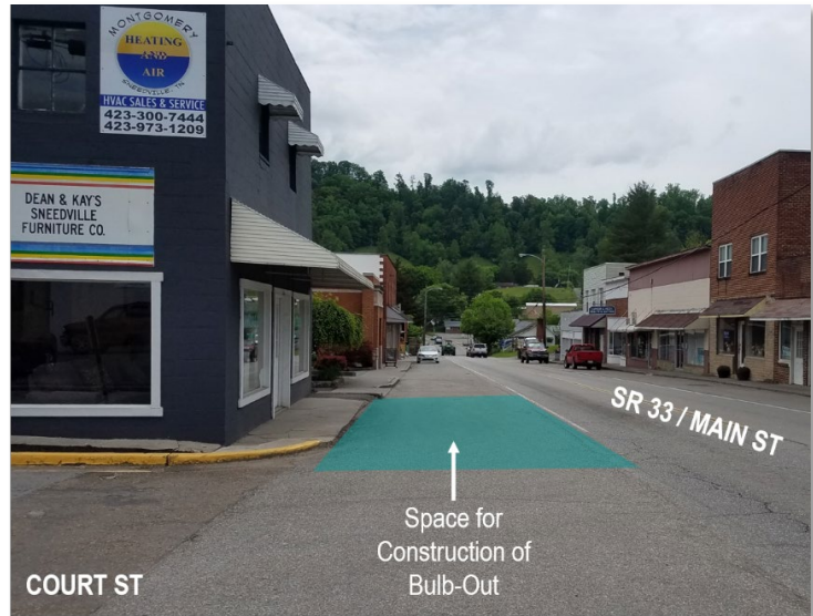
Looking westbound from the SR 33 / Main Street / Court Street intersection, this image shows the excess pavement space that could be utilized for the construction of bulb-outs at key intersections.
