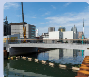
Bridge replacement work (Tobu Yachida Construction)
