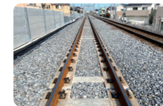
Ballasted ladder track
