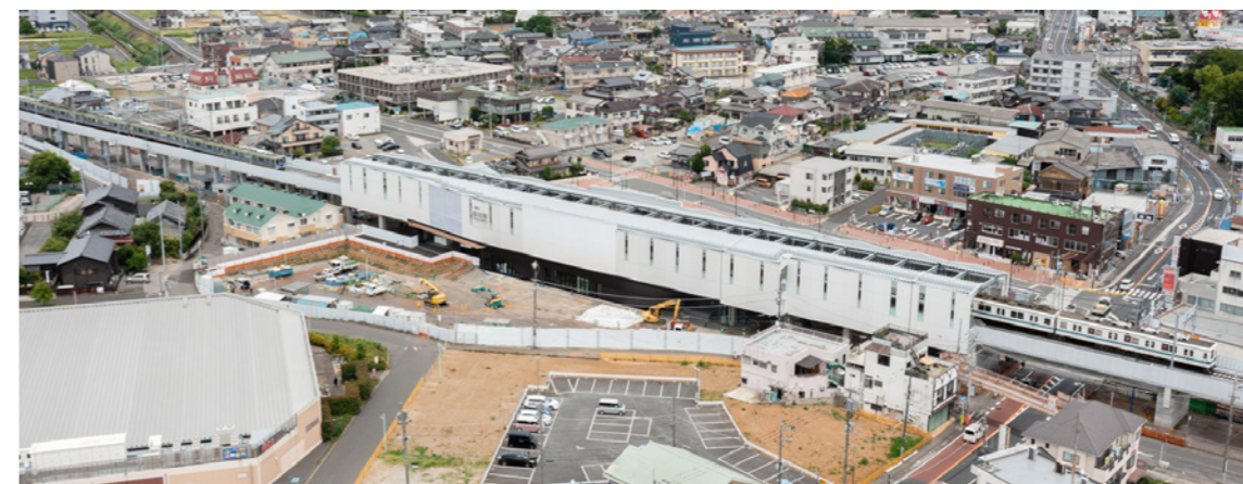
View near the elevated Atago Station
