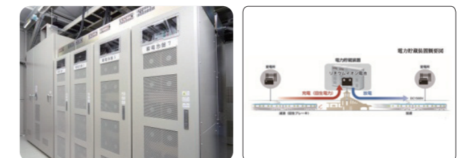
Regenerative power storage device
