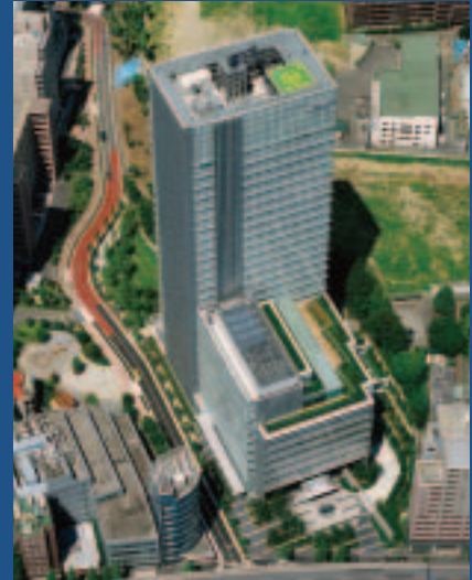
DNP Gotanda Building
