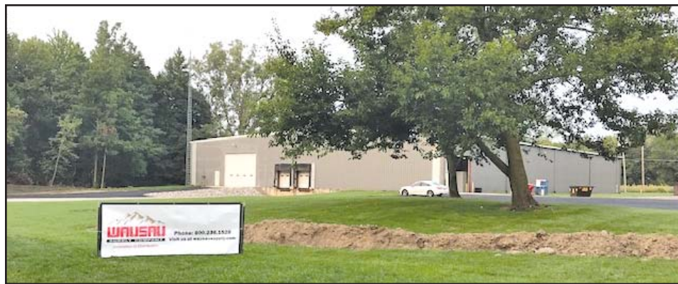
Wausau Supply is currently leasing a 30,000 square foot building in West Unity
