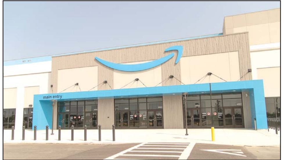
The front entrance of Amazon's new fulfillment center in Rossford
