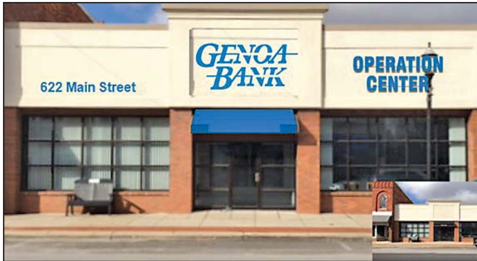
GenoaBank's Operations Center located at 622 Main Street in Genoa
