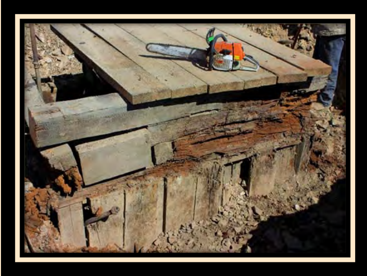
Damage to the wooden Silver Top mine collar.
