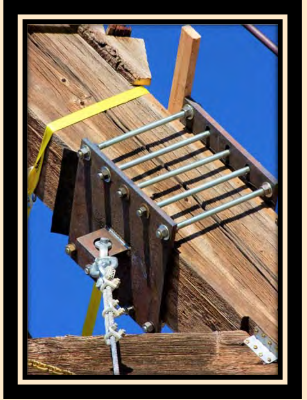
Metal support boxes were placed on the Silver Top Headframe for the crane to lift the structure.
