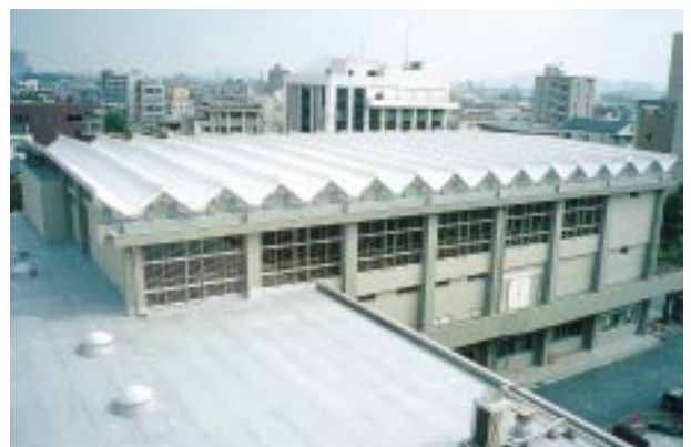
Torayca Lightroof* was used in this elementary school gymnasium built by Toray Construction Co., Ltd.
