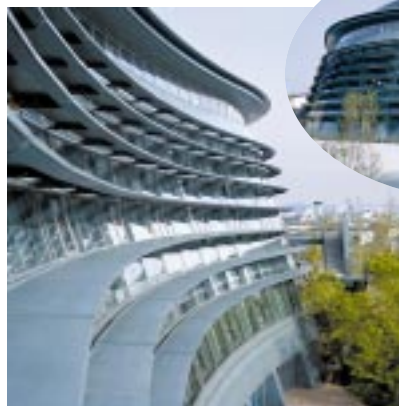
CFRP was chosen as a barrier for sunshine and rain in the Kyoto West Kyogoku Sports Center, which was completed in June 2002.
