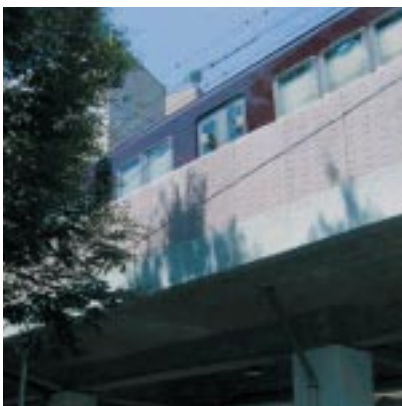
Toray's carbon fiber reinforced plastics (CFRPs) are used for soundproofing on an elevated railway line.
