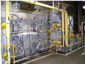
(the rebuilt boiler) | Fuel conversion for the in-house power generation boiler from <b>heavy oil to city gas</b><br>(Operation to start : July 2007)<br>
