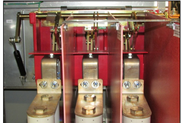
Fig. 23 Isolation Switch
