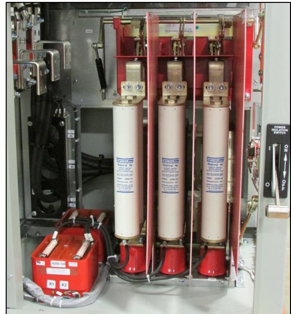
Fig. 22 Controller Compartment
