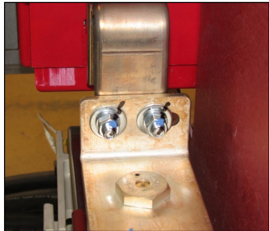
Fig. 42 Check Electrical Joints
