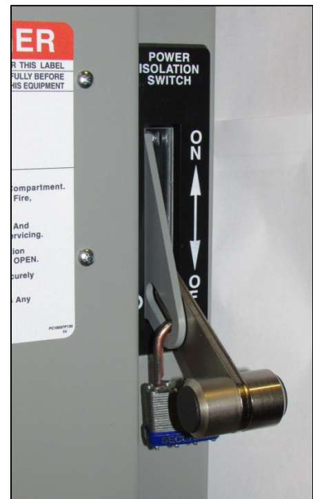
Fig. 24 Isolation Switch Lockout
