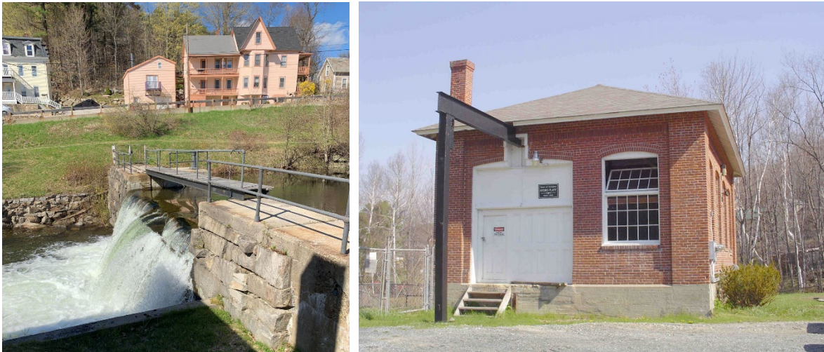
Photo 18. Historic 1840 granite block dam at River Rd, penstock in-flow for municipal hydro station and Town hydro-powered water pump. 2019 (left). Municipal hydro-electric generating station, next to town office (right). Credit: Barbara Chalmers.
