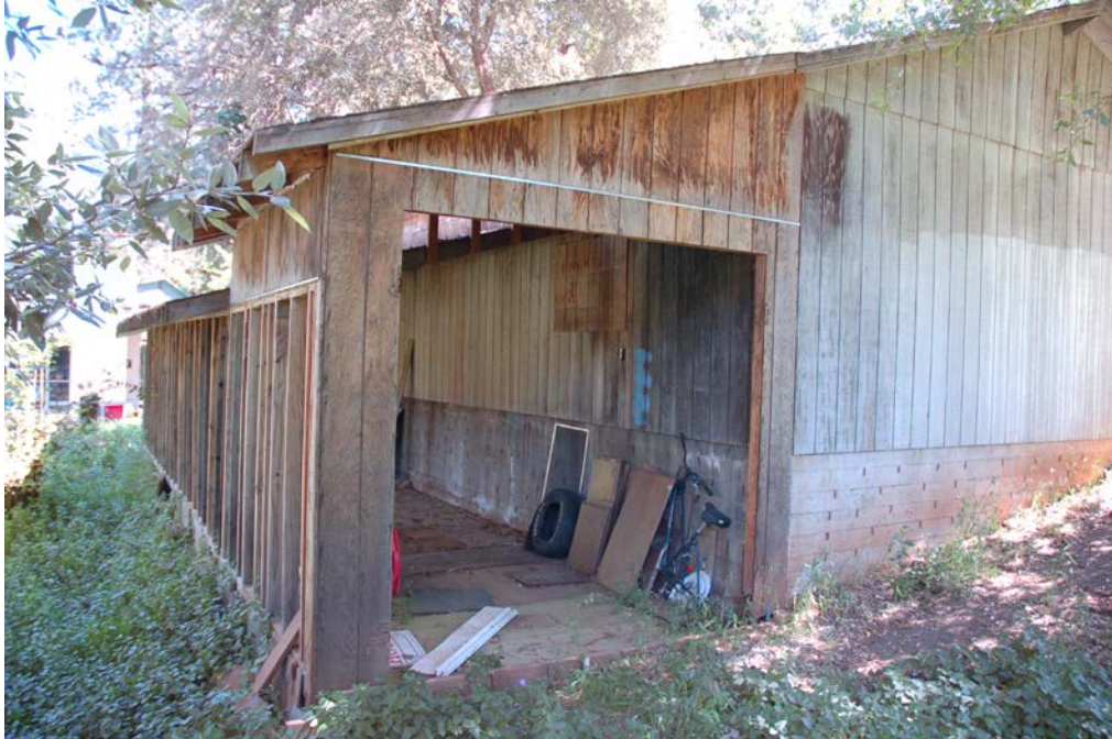
Photograph 4. View northeast of Building 2.
