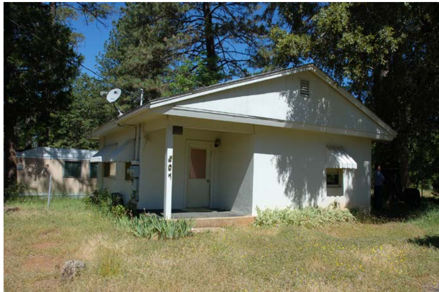
Photograph 5. View northwest of Building 5.
