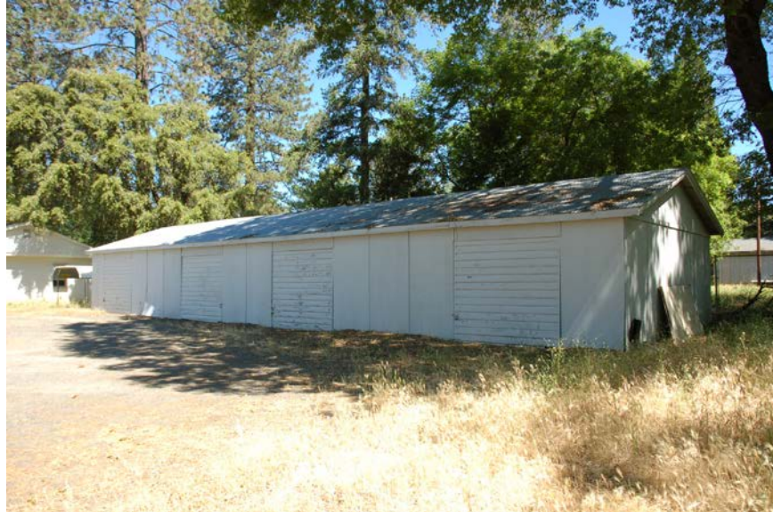
Photograph 4. View northwest of Building 3.
