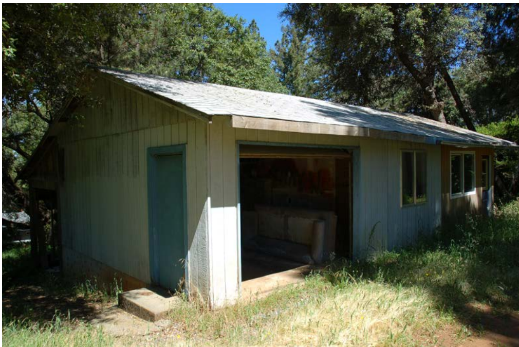
Photograph 3. View northwest of Building 2.
