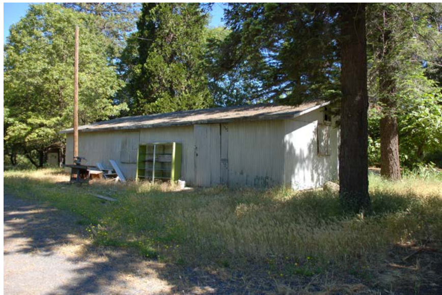
Photograph 3. View northwest of Building 2.
