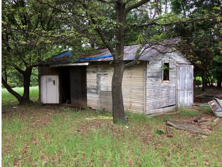
Photograph 4. View northwest of Building 3.
