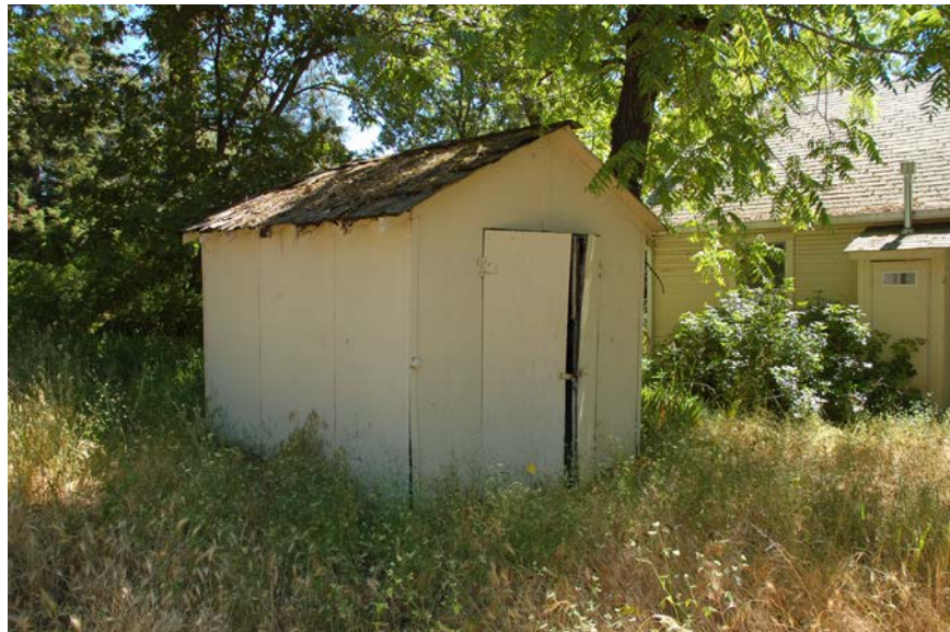
Photograph 7. View northeast of Building 9.
