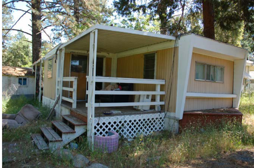
Photograph 6. View north of Buildings 6 and 7.
