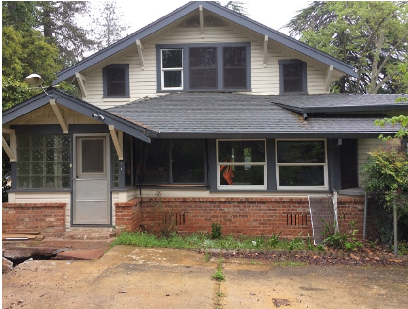
Photograph 2. View east of Building 1.
