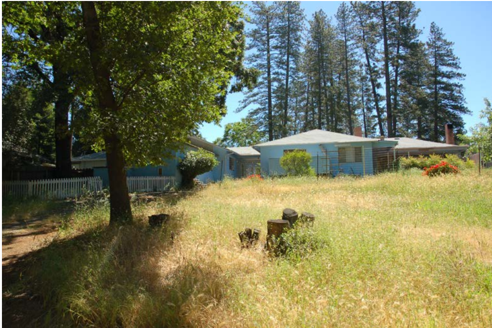
Photograph 2. View northeast of Building 1.
