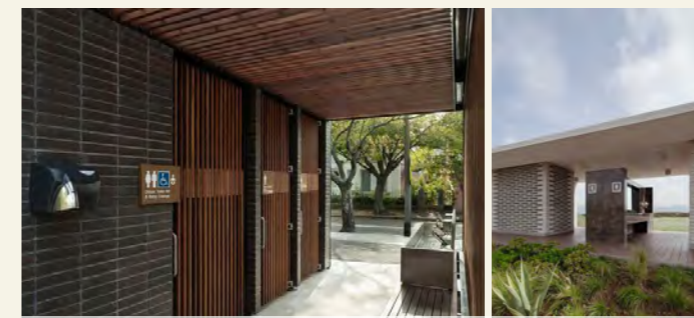
6 Constructing a new amenities block
