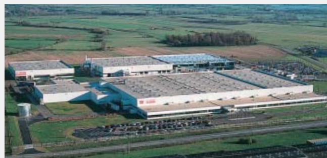
Toyota Industrial Equipment, S.A., our forklift truck production base in France, manufactures approximately 13,000 forklift trucks annually for the European market.
