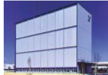
Rack Sorter BP Automated Storage and Retrieval System (Building Rack Type)
