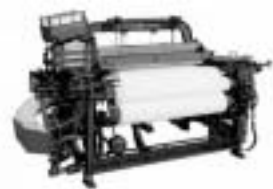
1924 Toyoda Automatic Loom Type G invented by Sakichi Toyoda.
