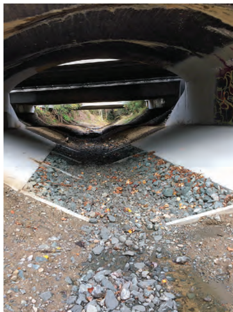
LEFT: The original fish ladder on Stevens Creek at the Evelyn Bridge. RIGHT: The completed creek bed and fish ladder before stream flow.
