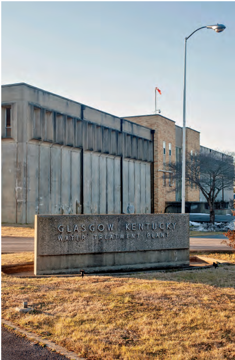
The Barren River Lake Water Treatment Plant was built in 1967 and expanded in 2007.
