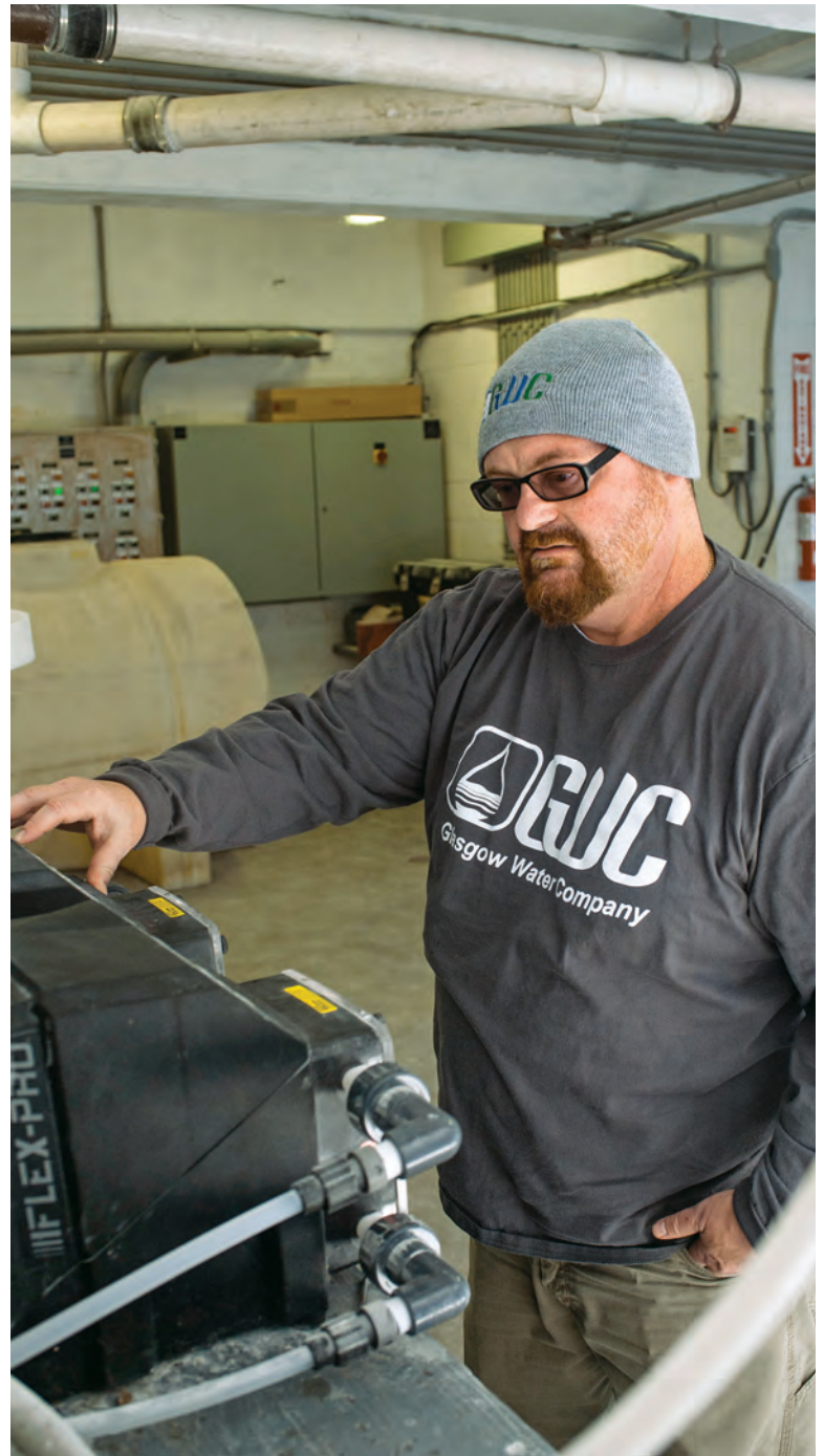
Scott Jones checks the coagulant feed.
