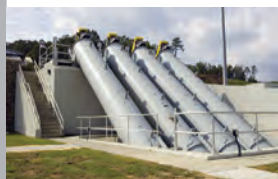
Tube-mounted screw pump from Schreiber
