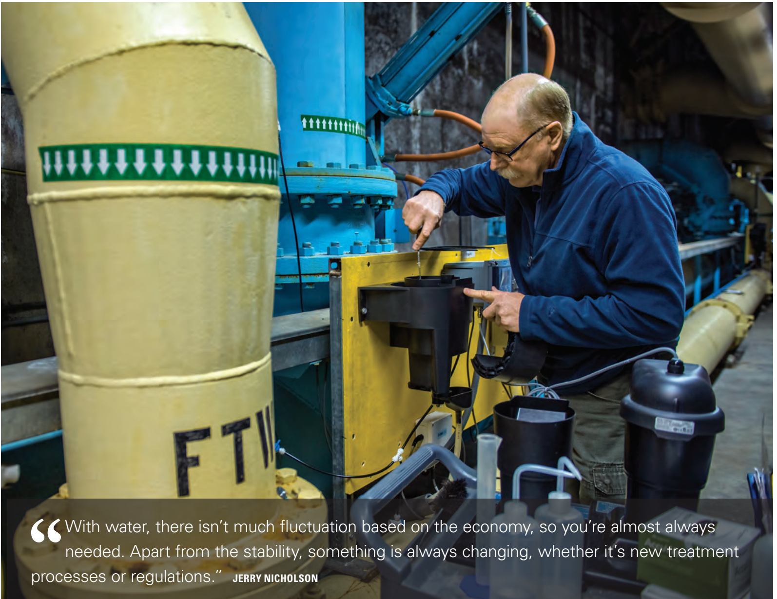
ABOVE: Nicholson cleans, verifies and calibrates a turbidimeter. LEFT: Valves release water from an indoor storage tank to outdoor storage ponds.
