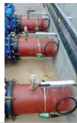
Flow Pulse flow monitor from Pulsar Process Management
