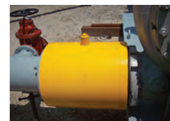
ProFlex Style 750 inline check valve from Proco Products
