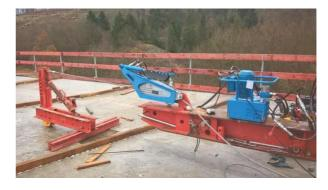
The Tirfor TU-A16 and TU-A32 can be motorized by a pneumatic system powered by an onsite or portable air supply and is operated by a standard control unit.
