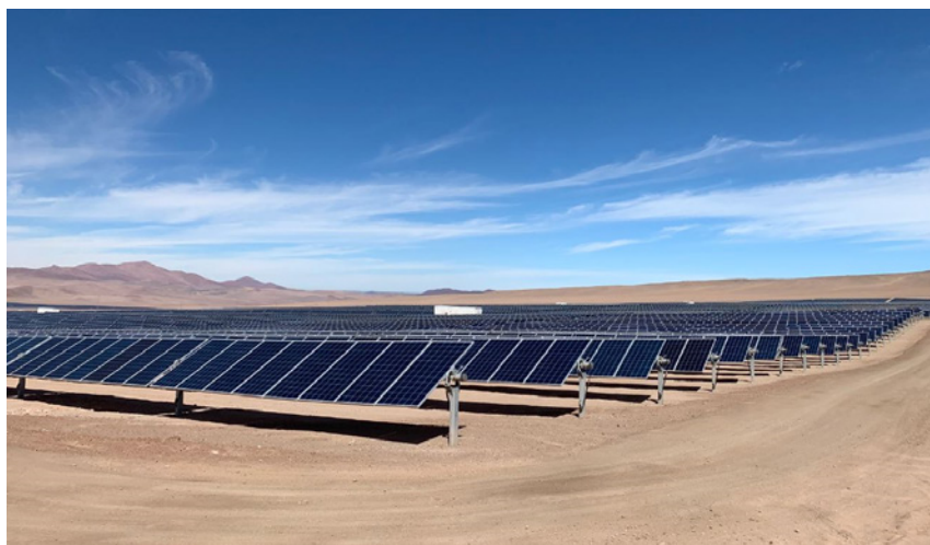
Construction of PMGD Photovoltaic Plant in Chile
