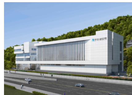
Construction of a Stable and Scalable Data Center
