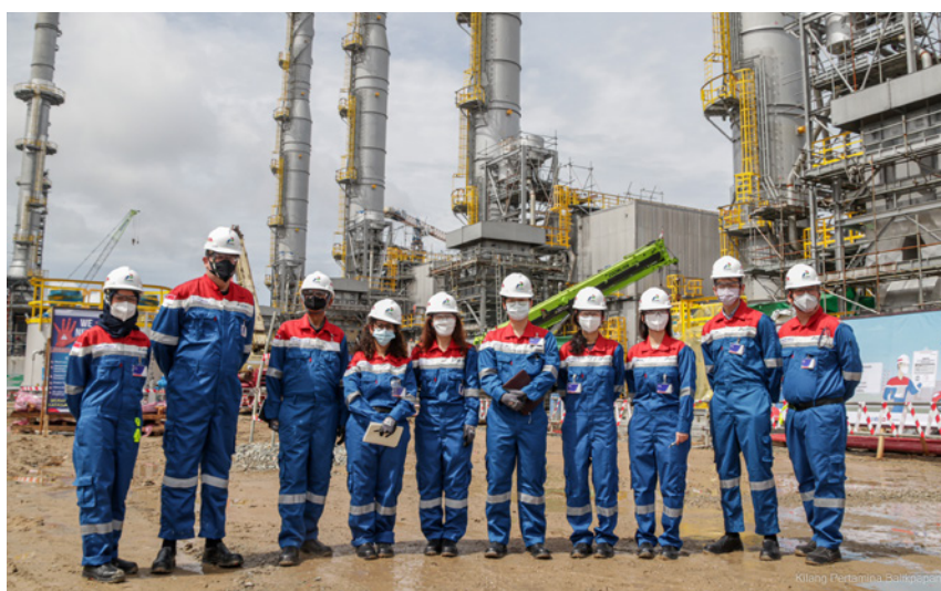
A site-visit for a refinery project in Indonesia
